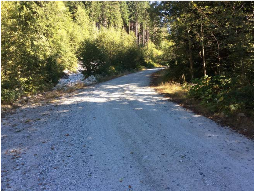
Left approach viewed from bridge
